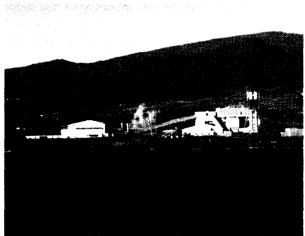
Distillery and power station (Réunion Island)
