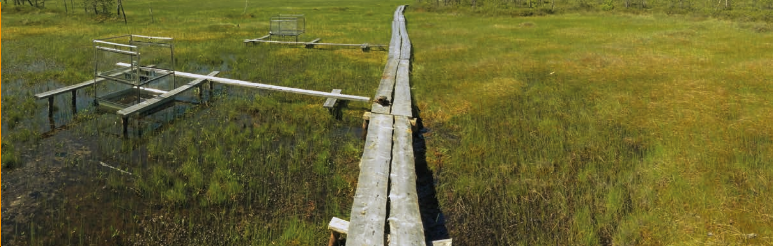
Boardwalks at Mukhrino Field Station to protect vulnerable vegetation (Wladimir Bleuten/Utrecht University).
