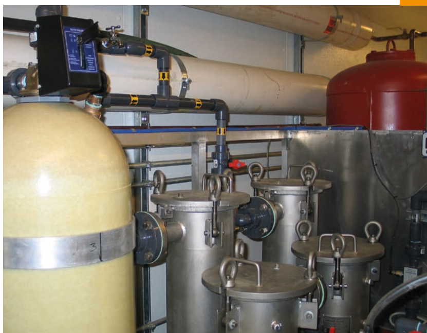
Filtering and other treatment of water is often necessary before use (Elmer Topp-Jørgensen/Aarhus University).
