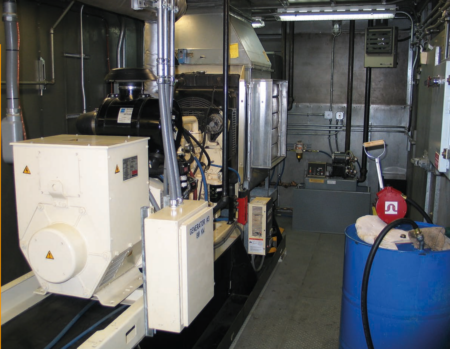
Generator providing heat and electricity for Toolik Field Station (Elmer Topp-Jørgensen/Aarhus University).
