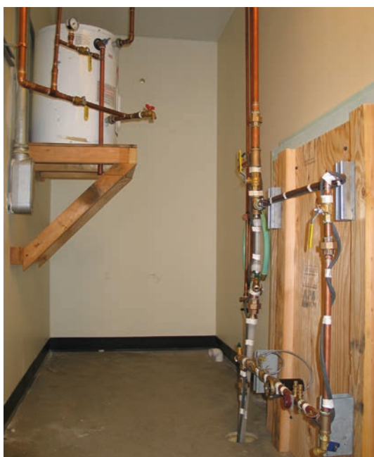
A circulation system can prevent water from freezing in tubes (Elmer Topp-Jørgensen/Aarhus University).
