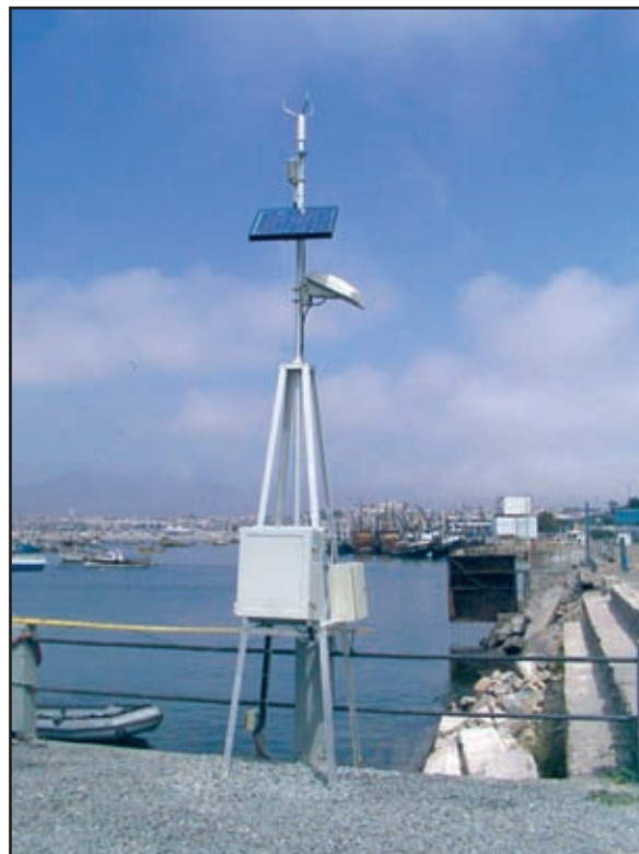
Figure 2. Sea level station configuration.
