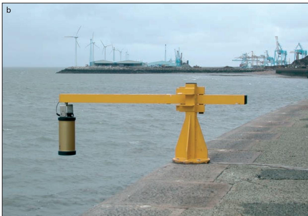
Figure 3.6 Radar tide gauges. (a) diagram comparing a radar and a bubbler gauge (Woodworth and Smith, 2003); (b) an OTT Kalesto test installation at Liverpool.
