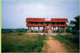
A cyclone shelter in Orissa, India
