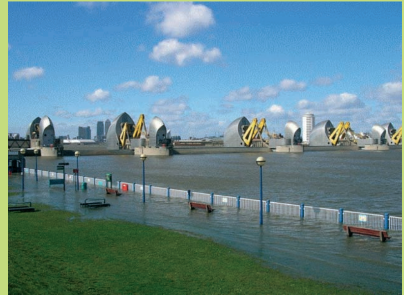
The Thames Barrier in operation – view upstream towards the city of London
