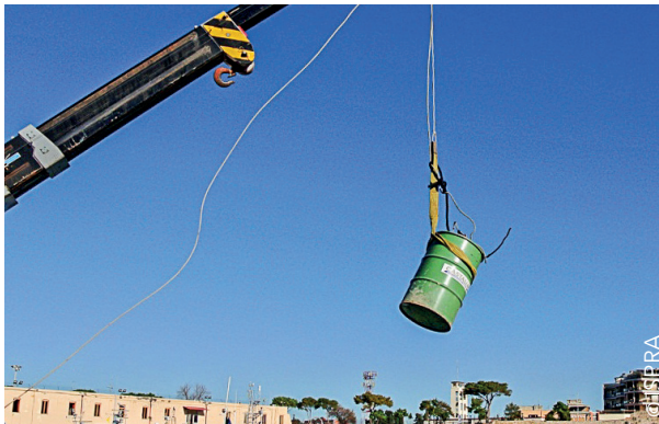
Lifting a drum with a crane
