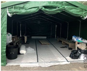
Example of worksite equipment
