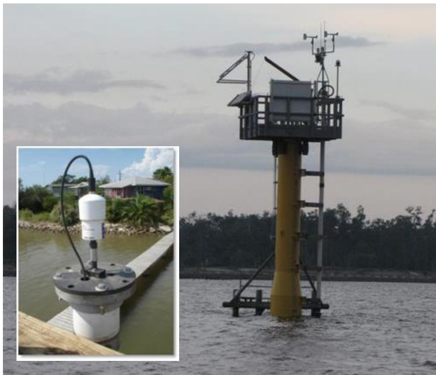
Figure 2-2. An elevated NOS/CO-OPS NWLON station using an Aquatrak acoustic WL sensor (inset) with a sounding tube housed inside a protective 6-inch PVC well.
