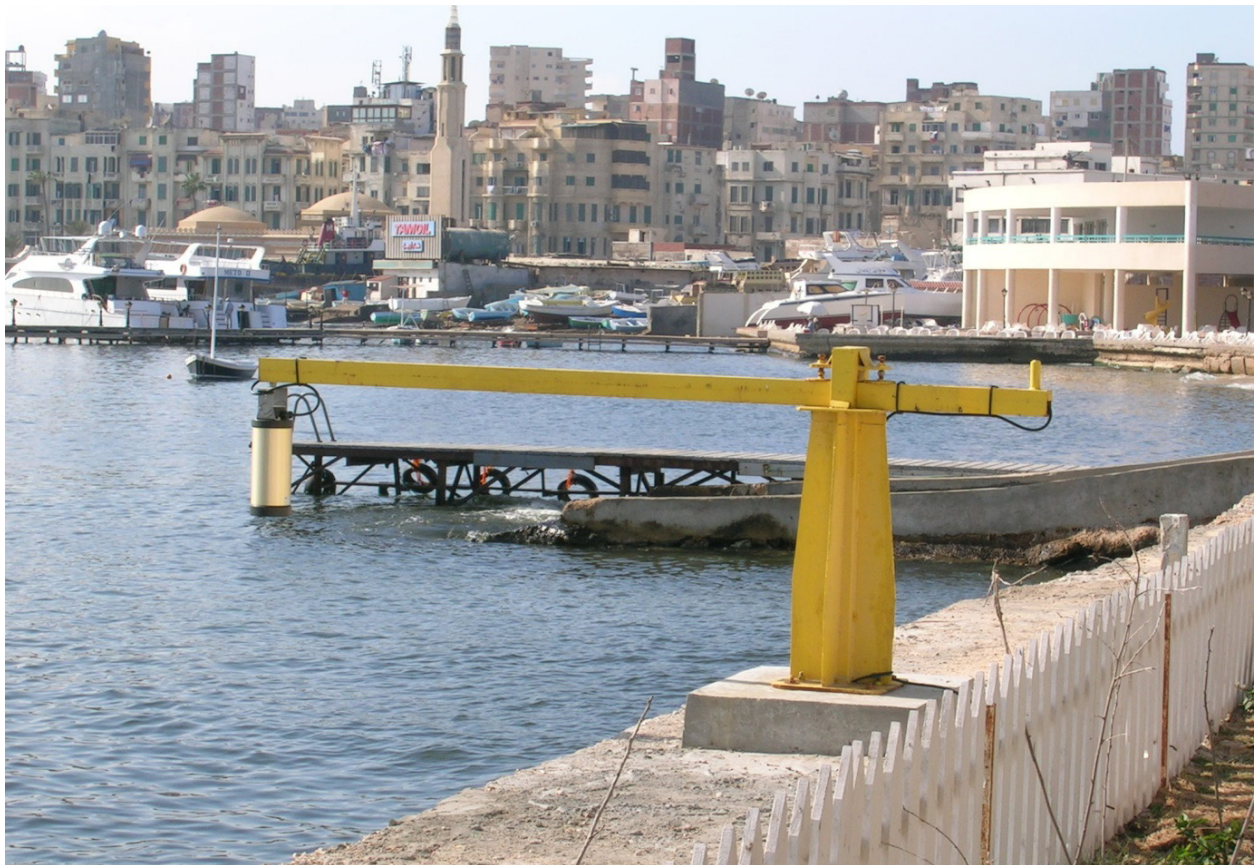
Figure 4.3 An OTT Kalesto gauge in Alexandria at the end of an arm that is pushed and bolted into place. (Photograph T. Aarup, IOC).
