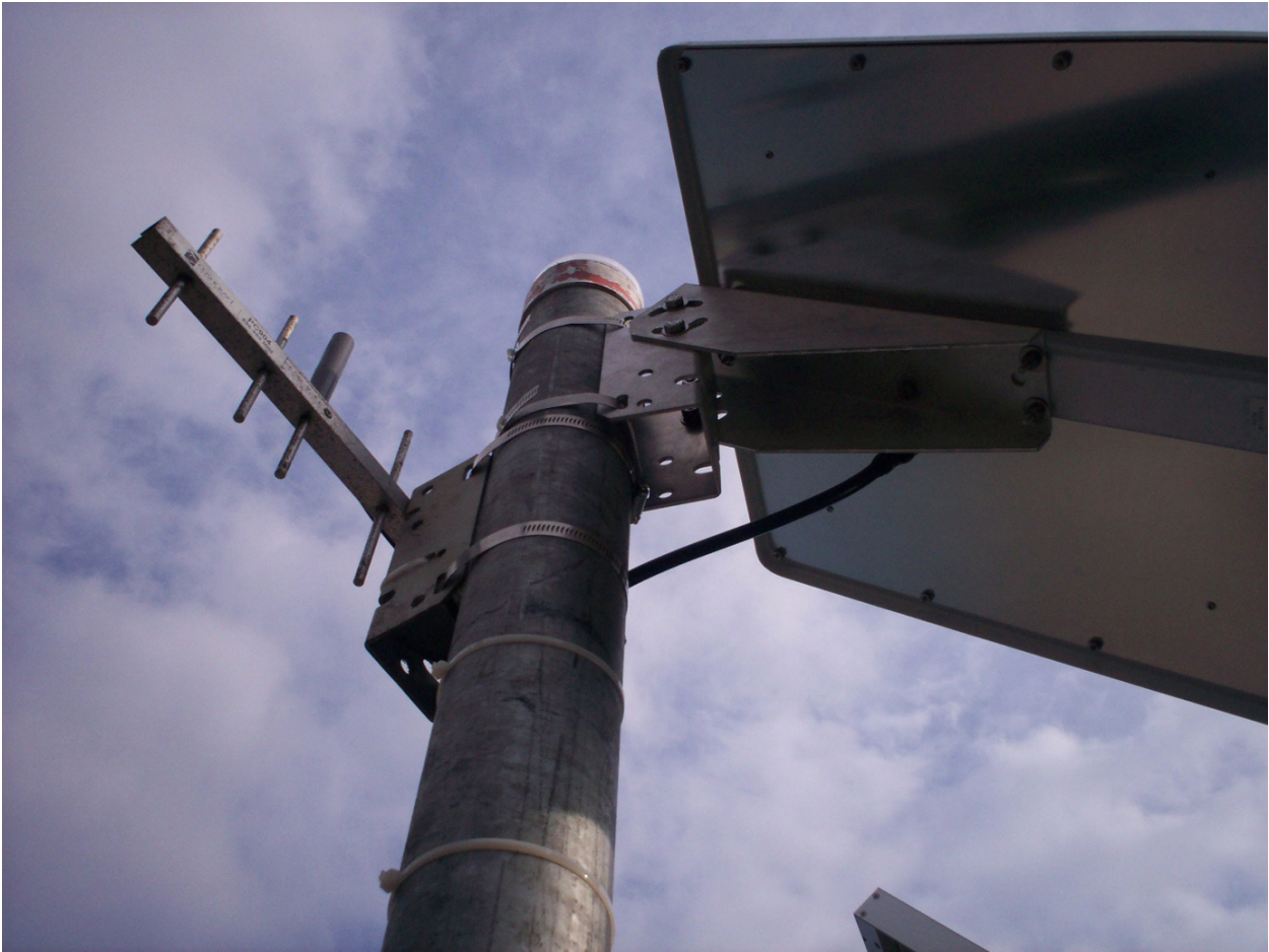
Figure 7.6 A compact local radio transmitter antenna at Antofagasta, Chile. (Photograph SHOA).
