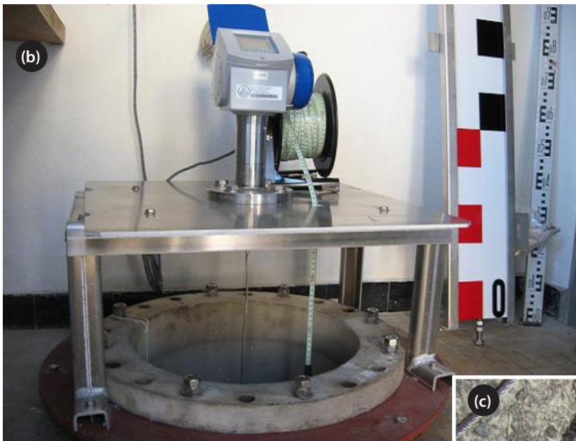
(b) A GWR sensor installed in an existing stilling well at Sète, France. (Photograph SHOM).
