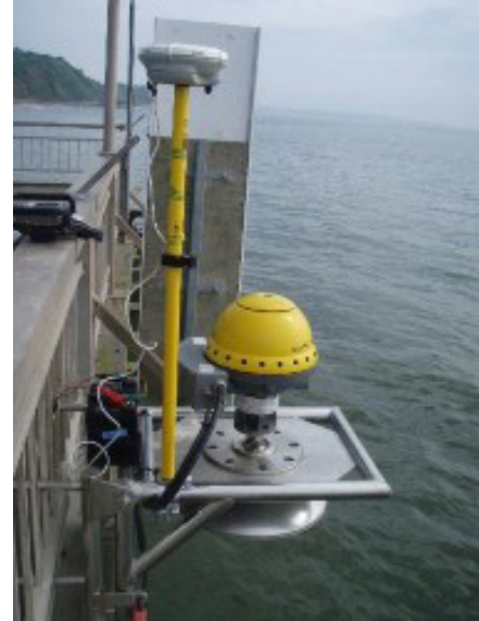
Figure 3. GPS survey of WaveRadar REX on Teignmouth Pier ©Teignbridge District Council.
