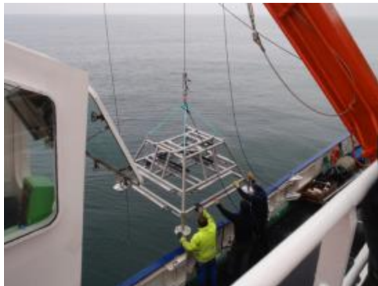
Figure 24. Deployment of new underwater elements with the ship crane.
