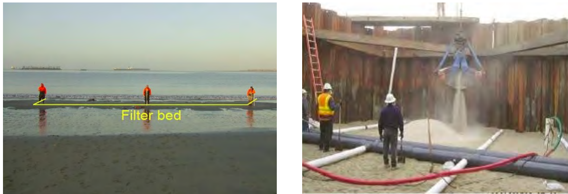
Figure 6.23. Filtration area of under-ocean floor seawater intake (left hand side) and filling of infiltration gallery with engineered sand during construction using a temporary cofferdam (right hand side) at Long Beach (Zhang et al. 2011). Reprinted with permission from American Water Works Association.
