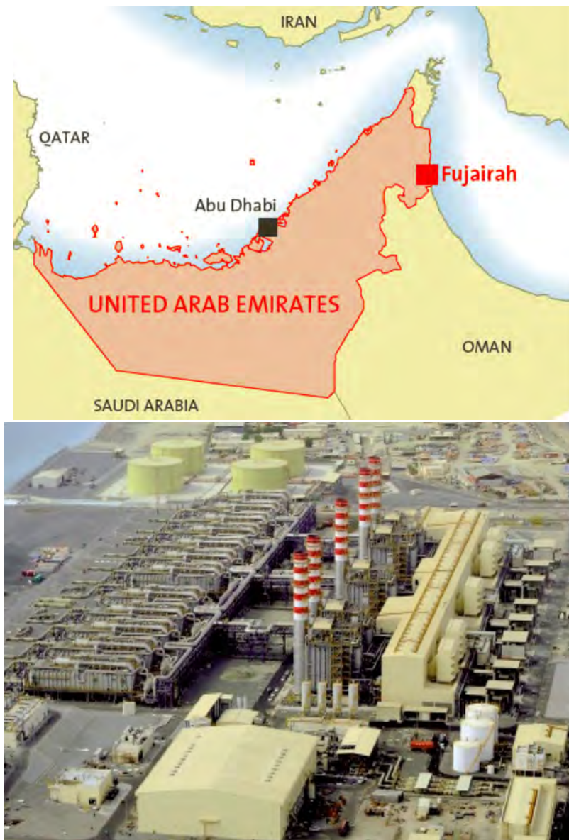
Figure 11.2.1. Location and aerial view of the Fujairah 2 hybrid plant in UAE. Photos: Veolia.
