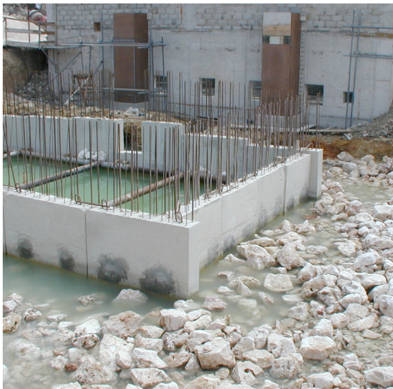
Figure 6.27. Karst pit intake system. Photo: T. Pankratz.
