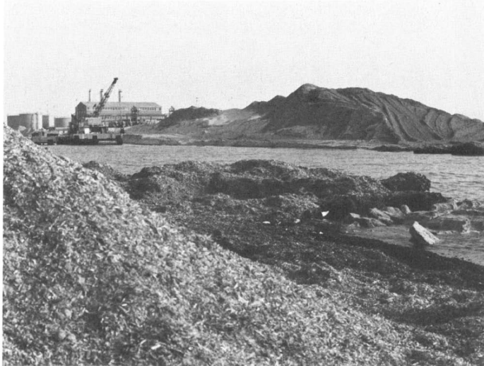
Figure 6.1. Dry seaweed extracted from the Zwitina desalination plant intake channel in Libya. Photo: Kershman 1985.
