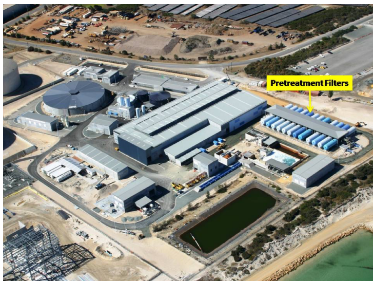
Figure 9.23. Single-stage horizontal -pressure dual media filters at the Kwinana SWRO Plant. Photo: Water Corporation.
