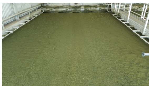
Figure 9.17. DAF float layer when treating a cyanobacterial bloom. South Australian Water Corporation Bolivar WWTP DAFF plant. Photo: Biomass lab, UNSW and SA Water.
