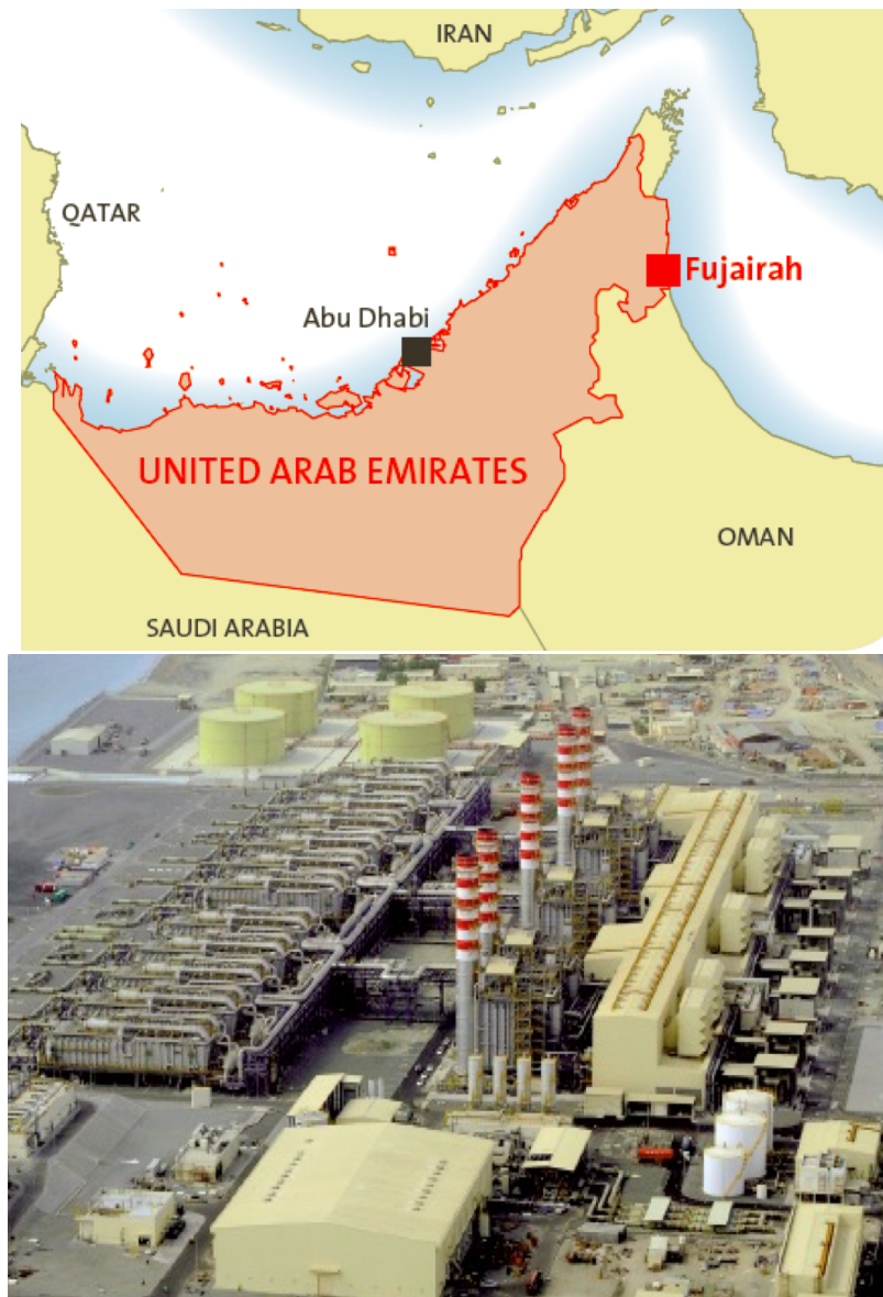
Figure 11.2.1. Location and aerial view of the Fujairah 2 hybrid plant in UAE. Photos: Veolia.
