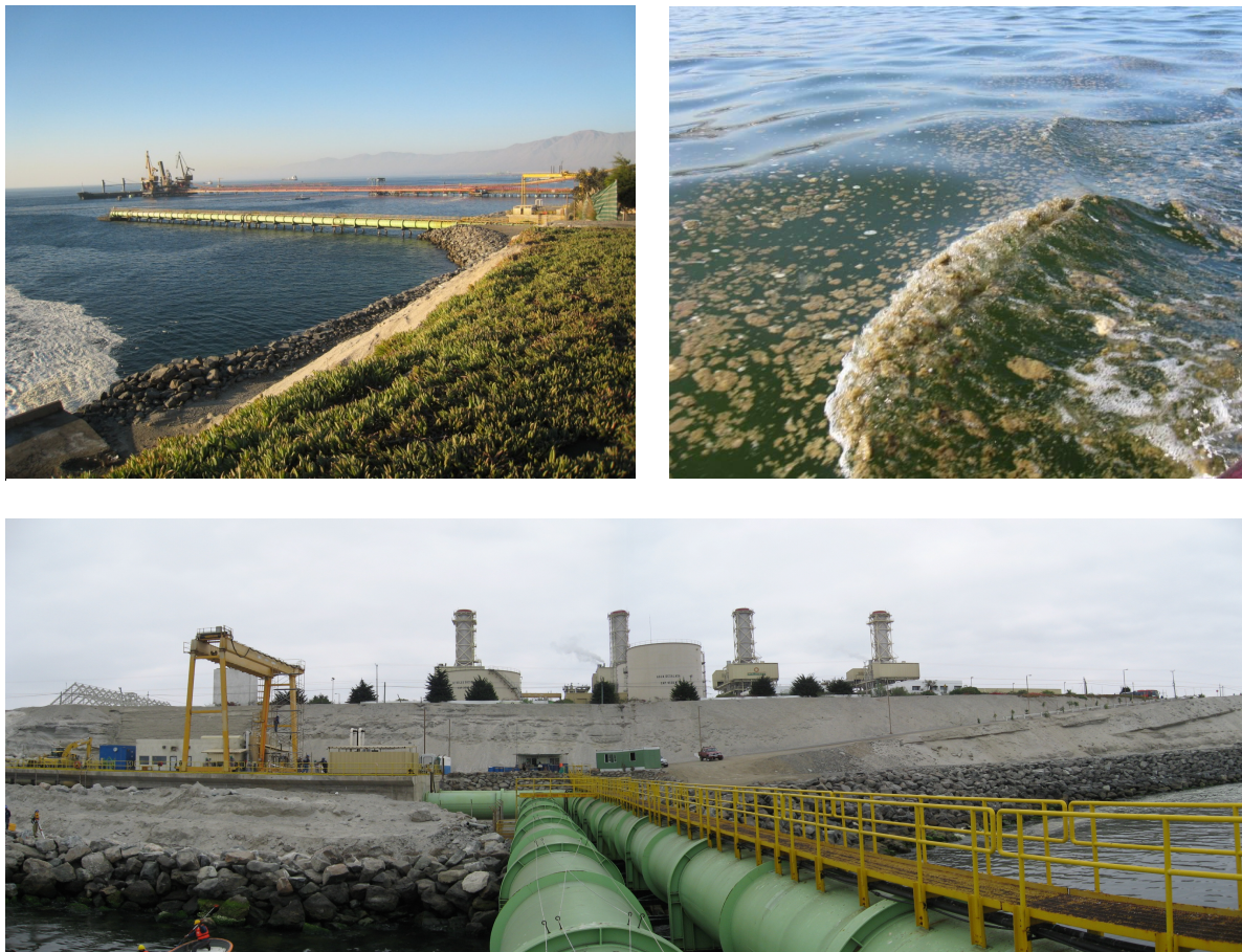
Figure 11.7.1. Intake to the Gas Atacama SWRO Plant (top left and bottom) and the algal bloom discussed in this case study. Bloom photo: Aquacien Consultoria Maritima.
