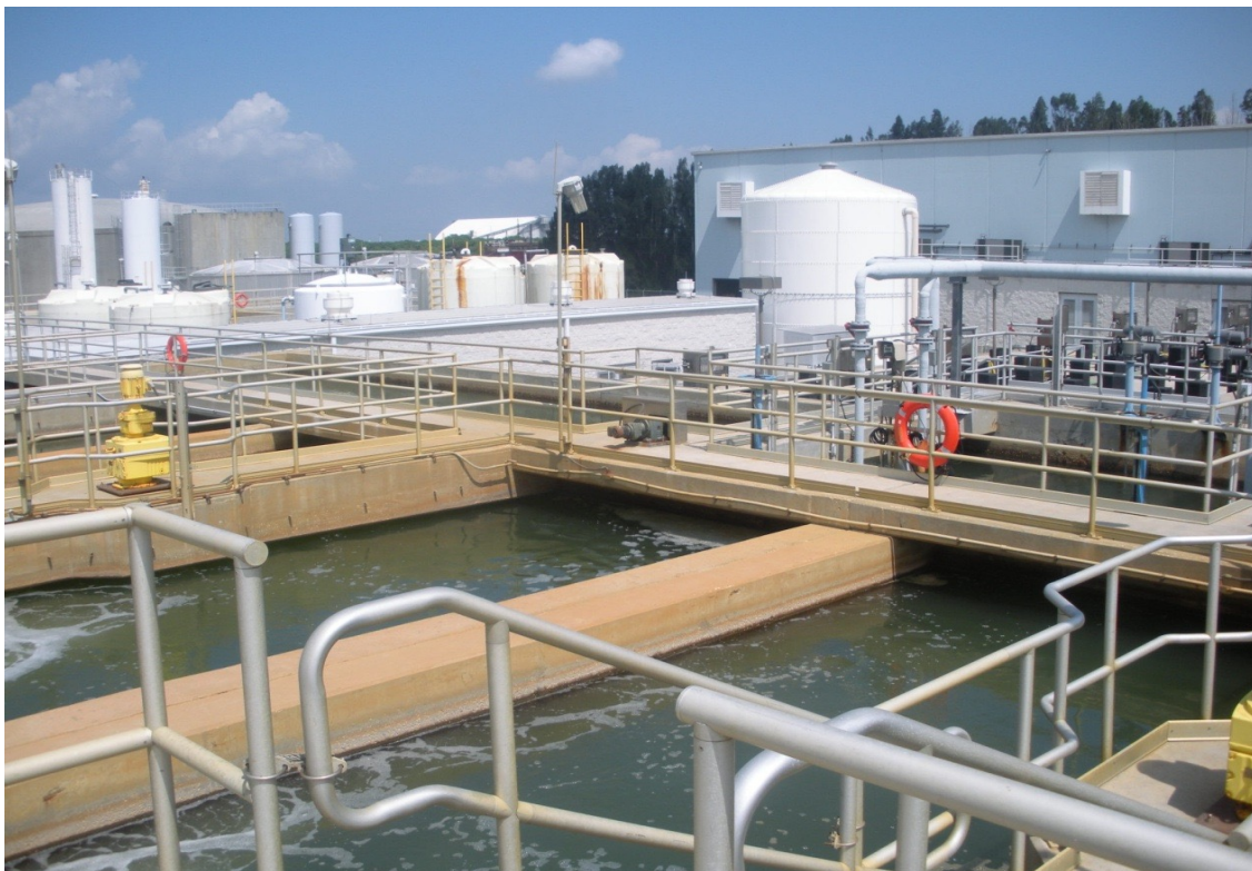
Figure 11.9.3. Normal pretreatment basin appearance (Voutchkov 2009).
