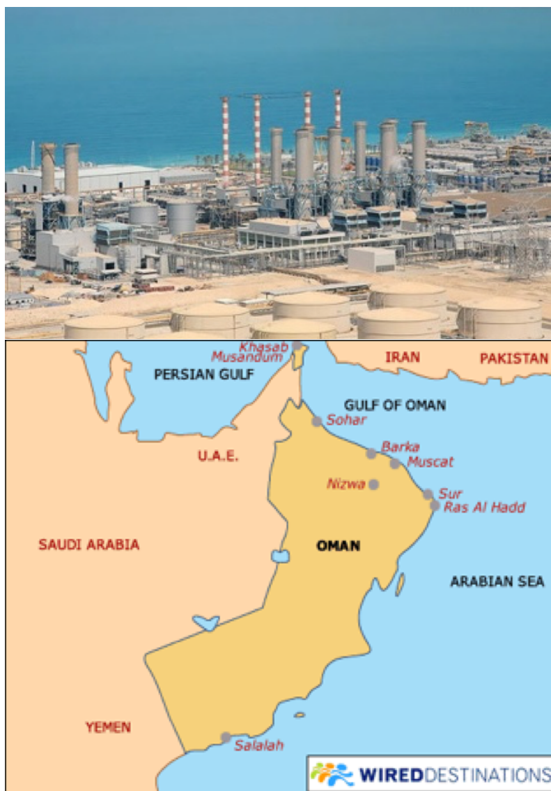
Figure 11.4.1. Location and aerial view of Barka 1 desalination plant in Oman.
