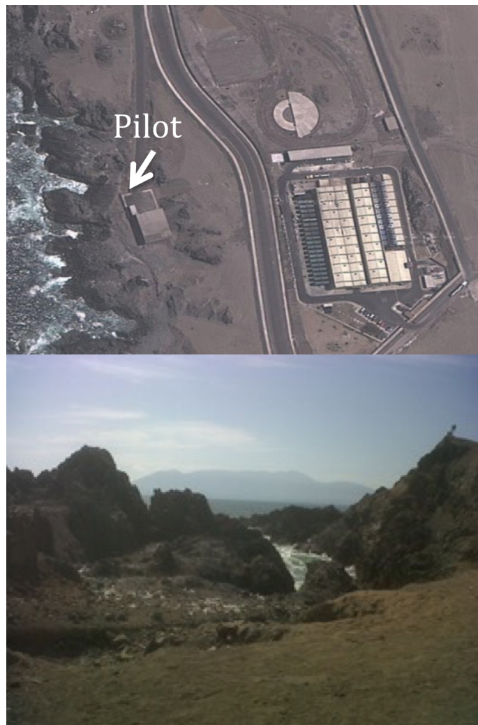
Figure 11.8.1. Aerial photo of pilot plant area at La Chimba Antofagasta (top). Photo: Google Earth). Intake area of the pilot plant (bottom). Photo: Abengoa.
