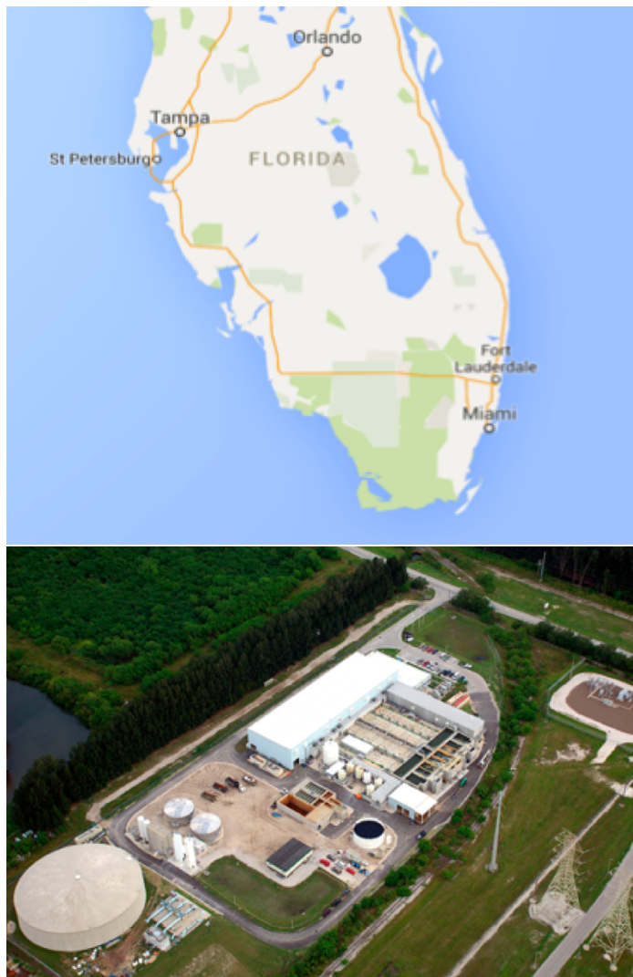
Figure 11.9.1. Location of the Tampa Bay Seawater Desalination Plant (top) and aerial view (bottom; Accessed on 11 Nov. 2016 http://www.accionia.us/projects/water/desalination-plants/tampa-bay-desalination-plant/ ).
