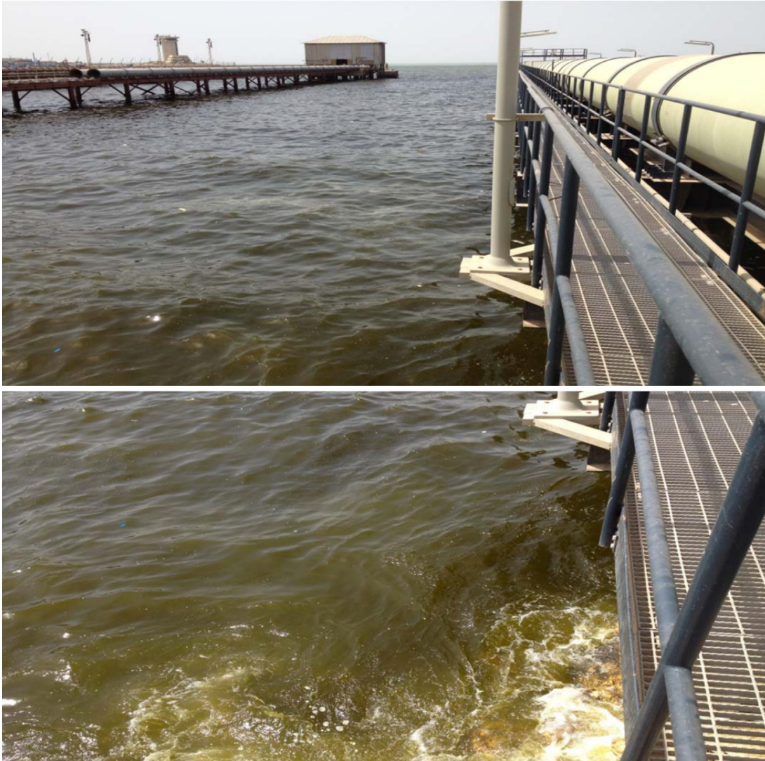
Figure 11.5.5. Seawater conditions during the algal bloom (top) showing the condition of the seawater close to shore (intake pipe at right of image); bottom shows a close-up of the green-brown hue produced by the algae.
