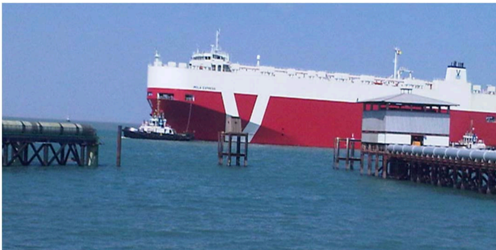
Figure 11.5.4. Shipping traffic passing by the Shuwaikh intake (pictured at left), heading into the Shuwaikh Port (left and out of frame).
