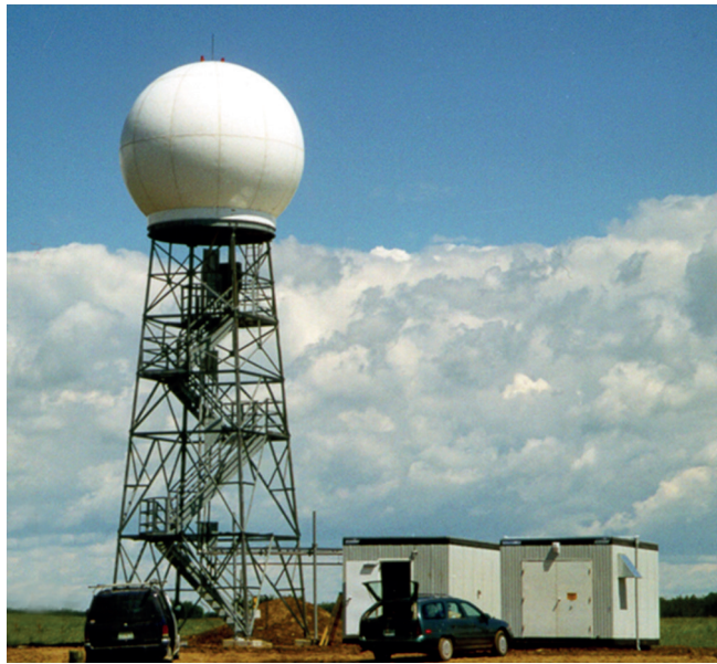
Figure 7.1. A typical weather radar within the Canadian network showing the major physical components of a radar system. The tower is about 30 m high, with a radome fitted with hazard lights and a lightning rod.
