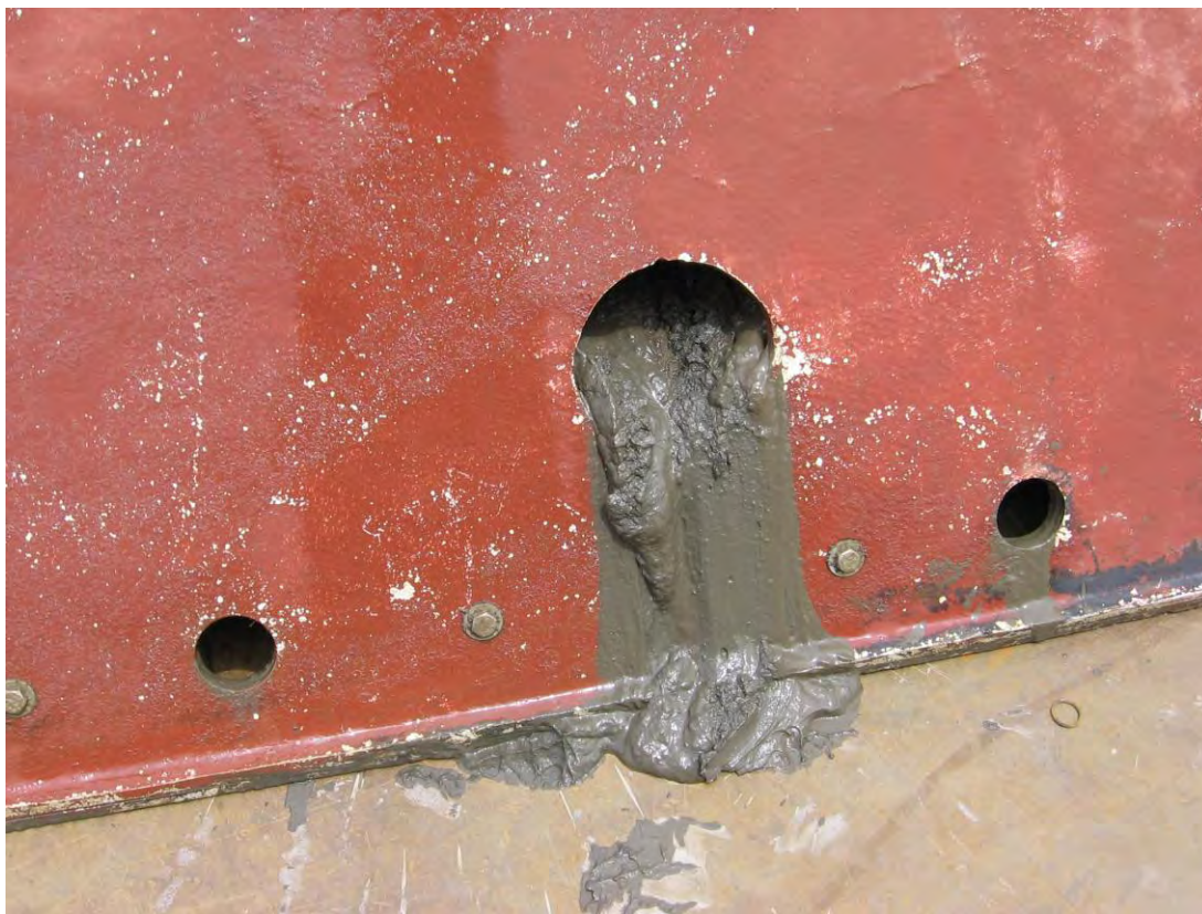
Figure 11. Sedimentation inside the ES II
