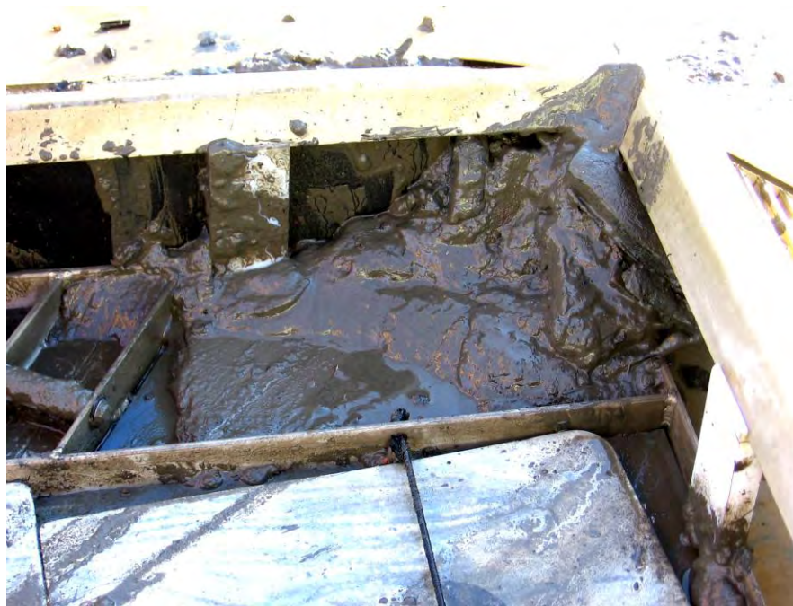
Figure 12. Sedimentation inside the base of the TRBM. Note that some silt has been washed away when the base is lifted up through the water column.
